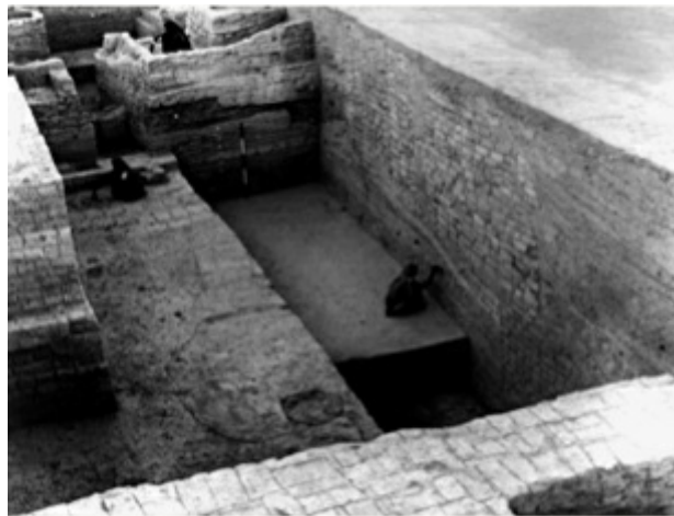
CROSS-SECTION OF DEFENCE WALL
